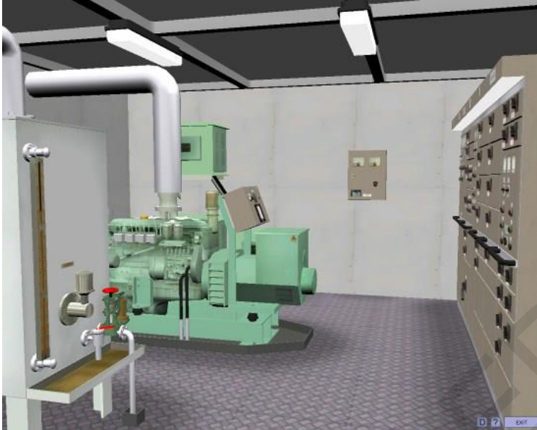
Fig. 41 Emergency generator
