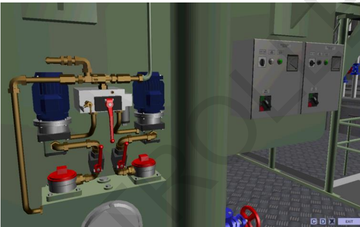
Fig. 27 Alfa Cylinder Lubricating Oil System
