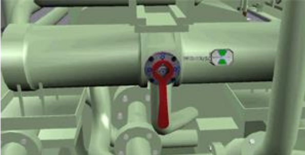
Fig. 26 Filter's contamination indicator DG
