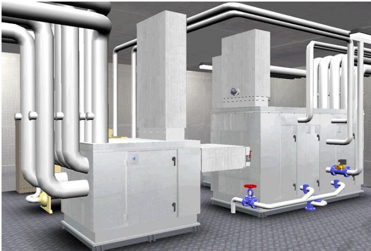
Fig. 73 Air Handling Unit
