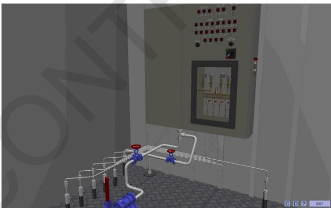
Fig. 91 Quick Closing Valves Release Station
