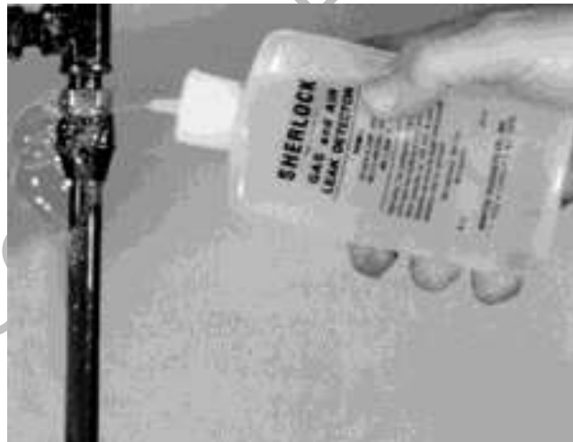
A simple bubble test for leak detection.
